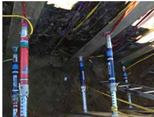
Here is a completed system.
