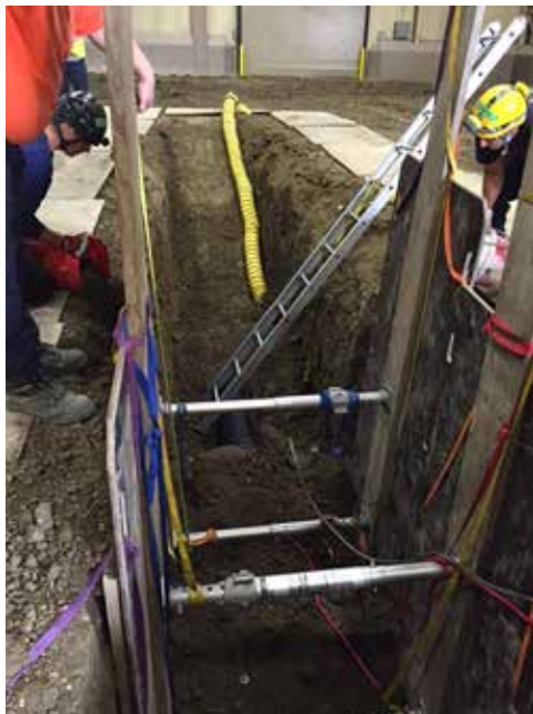
Students have panels in place to complete box. Backfilling behind panels before struts are shot to full pressure.
