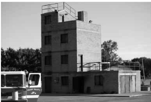
Cherry Valley live-fire training tower
