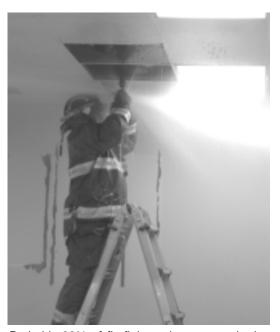
Probably 99% of firefighters have never had to plug a charged sprinkler head. During this training, they experienced problems in inserting the plug to stop the water flow because of pressure.
