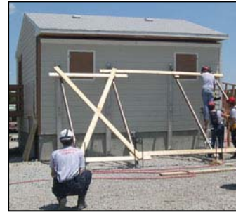
Structural Collapse Rescue Training
